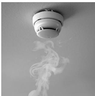
Inside the smoke detector a radioactive source causes ionisation of the air between two electrically charged plates. When smoke enters the detector, the ionisation of the air is reduced.
